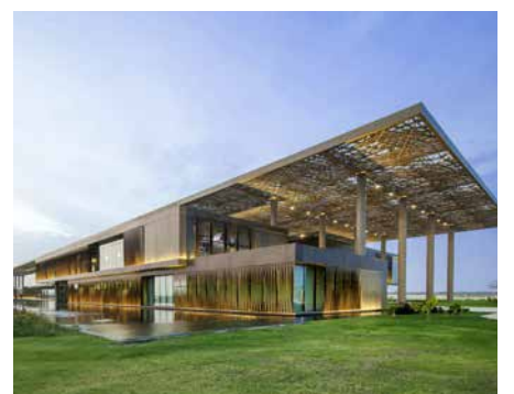
Data Center Senegal
